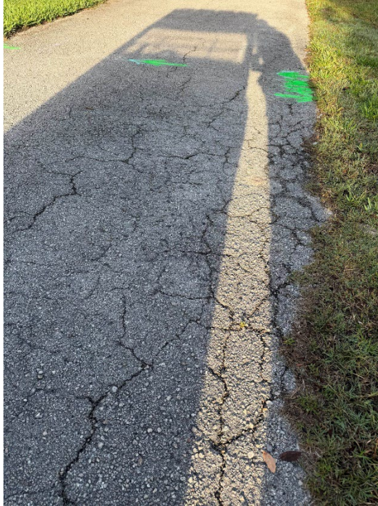
Photo 6.1 – Typical Asphalt Raveling and Base Failure (New Photo – 2026 Assessment)
