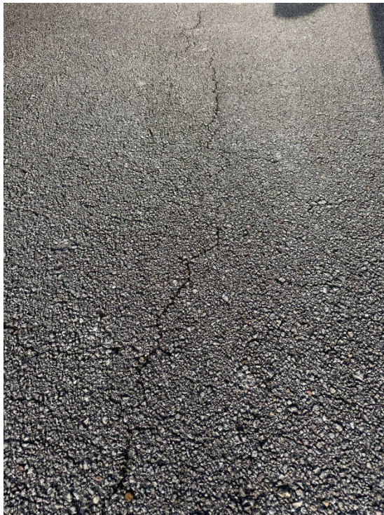
Photo 7 – Typical Asphalt Raveling (No Observed Changes) (Refer to Prior Photos 8 and 9– 2025 Assessment)
