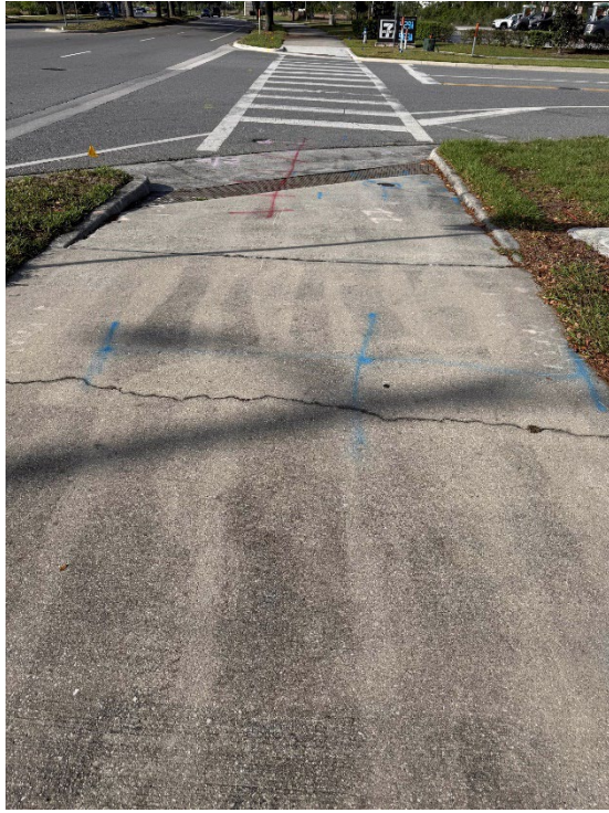
Photo 18 – Surficial Cracked Concrete (No Observed Changes) (Refer to Prior Photo 25 - 2025 Assessment)
