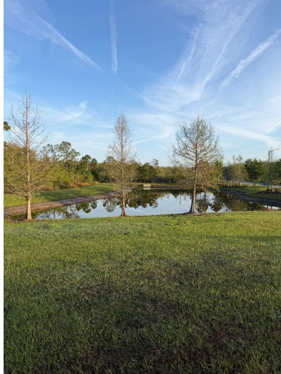
Photo 1 – Wellspring Drive Pond SMA-WD in Good Condition (No Observed Changes) (Refer to Prior Photo 1 - 2025 Assessment)
