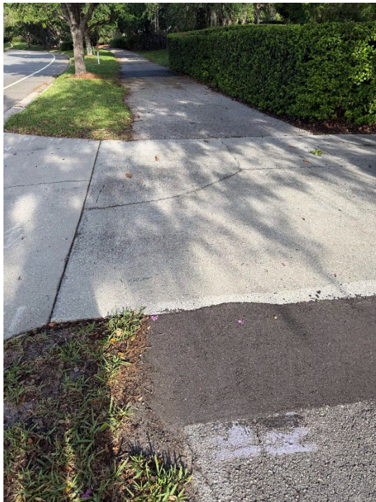
Photo 16 – Surficial Concrete Cracked in Driveway Apron (No Observed Changes) (Refer to Prior Photo 20 - 2025 Assessment)
