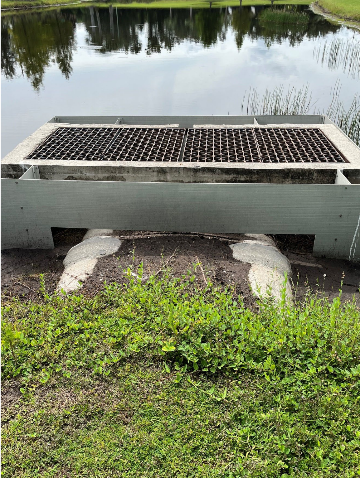
Photo 4 – Water Control Structure in Good Condition
