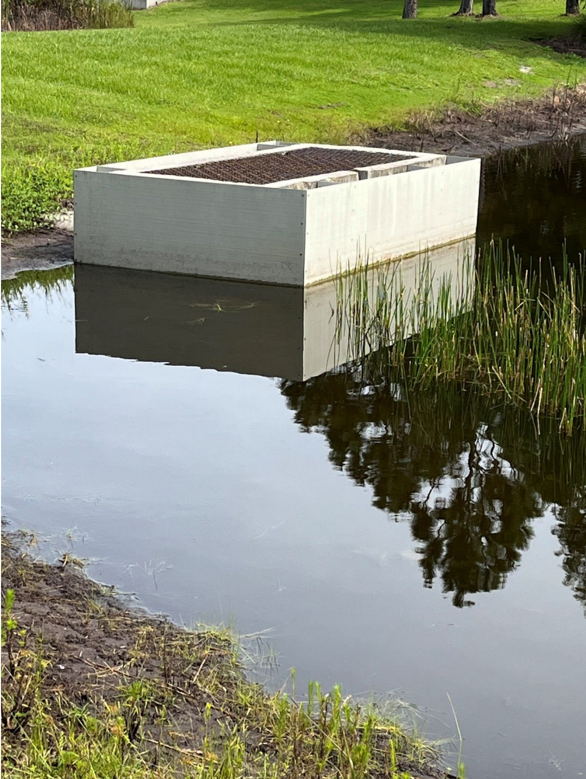
Photo 2 – Water Control Structure in Good Condition
