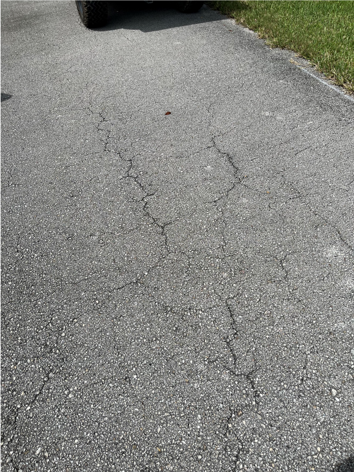
Photo 9 - Asphalt Raveling
