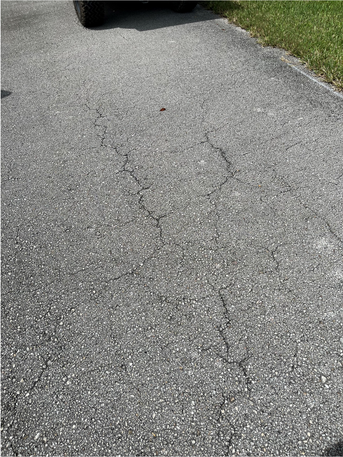
Photo 9 - Asphalt Raveling
