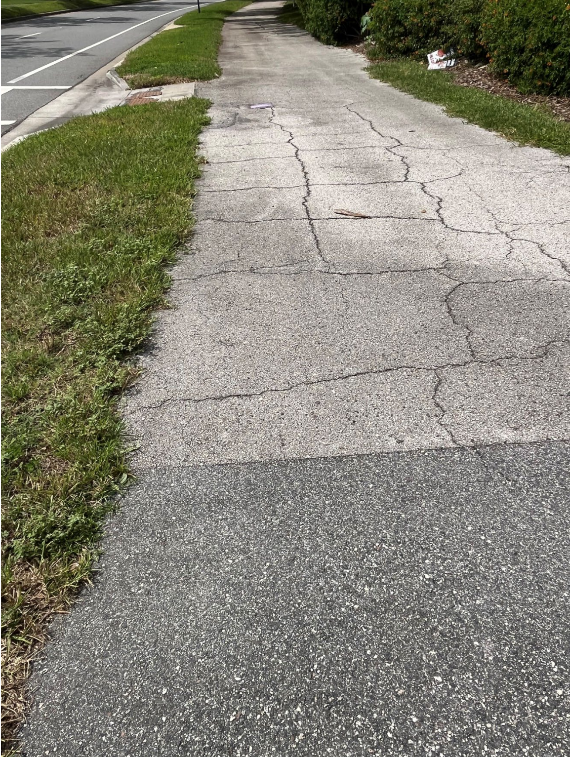
Photo 21 – Alligator Cracking
