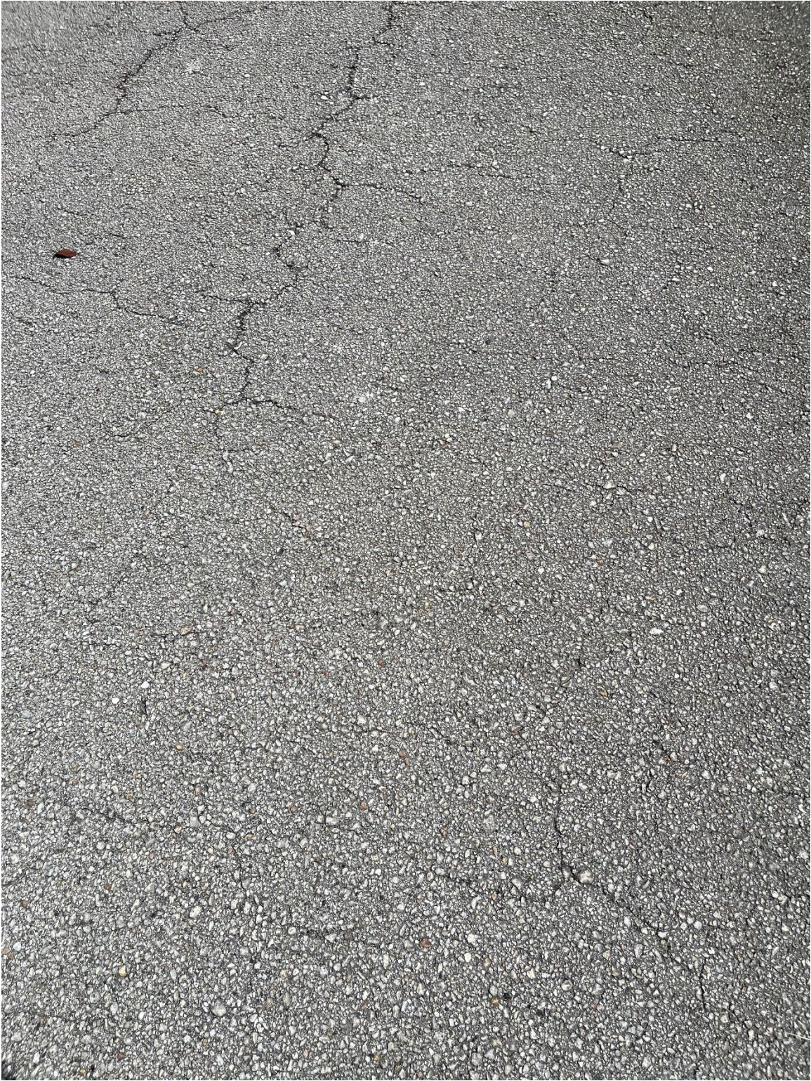
Photo 8 - Asphalt Raveling
