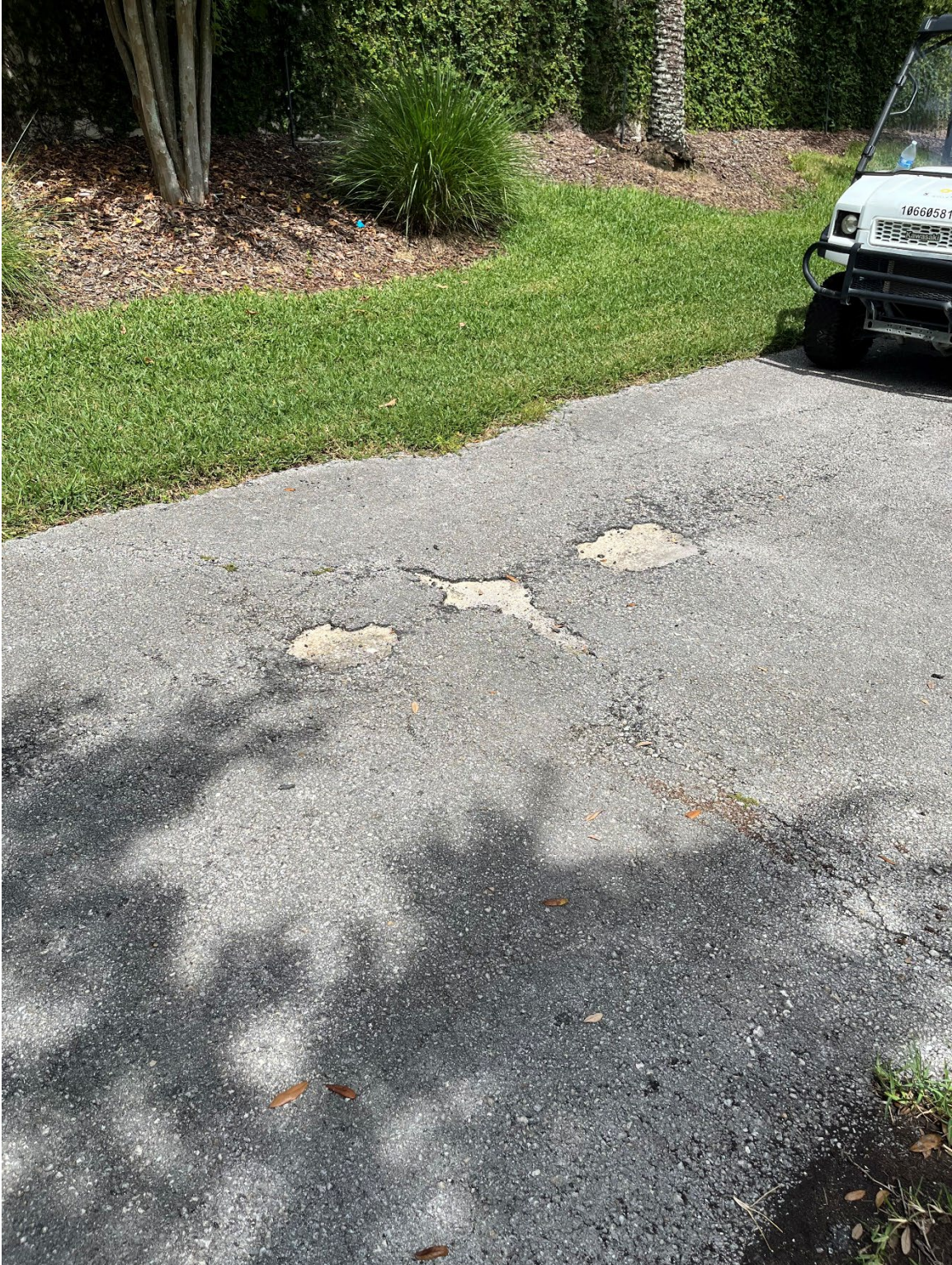
Photo 12 – Asphalt Damage
