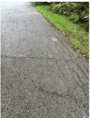
Comments Along the trail, it was noticeable that many tree roots were growing through the bottom of the asphalt. As a result, the pathway now bevels and is uneven, which poses a few challenges for those using the trails. Within the area, we now have standing water as a result of uneven surface area.
